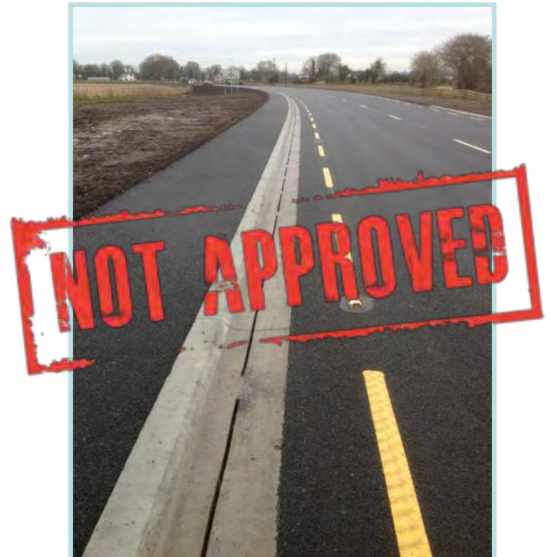
Nearside linear drainage channels.
