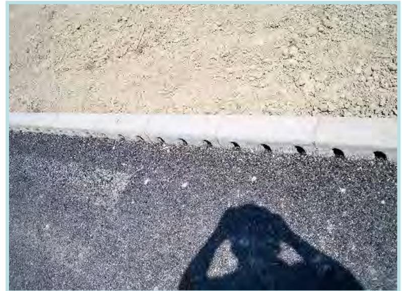
Example of combined kerb and drainage system on M3/N3 Clonee to Kells.
