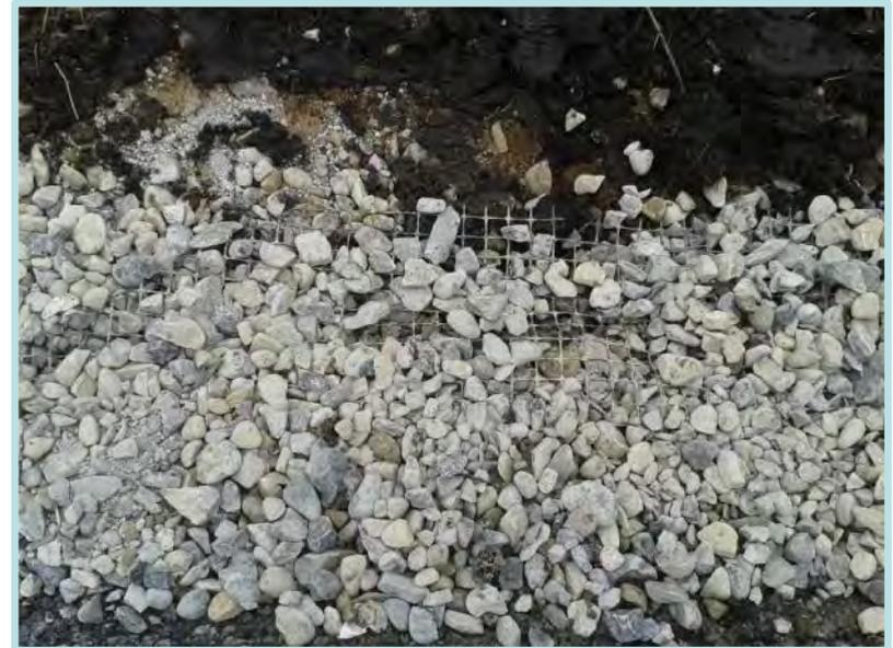
Surface of combined filter drain with geogrid.
