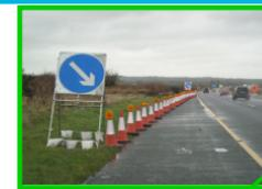
Rotating reflectors may be used in place of steady state lamps on the longitudinal sections of cones or barriers adjacent to the trafficked edge but may not be used on lead in tapers.
