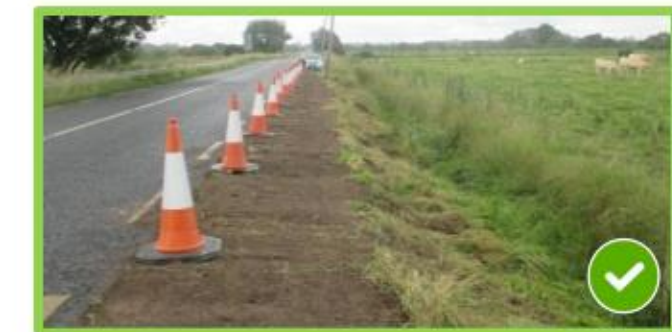
Figure 5.14 - Verge re-profiling works carried out prior to VRS installation
