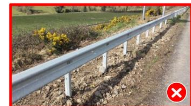
Figure 5.16 - Poorly reinstated following VRS repair works – uneven, large stones, not seeded
