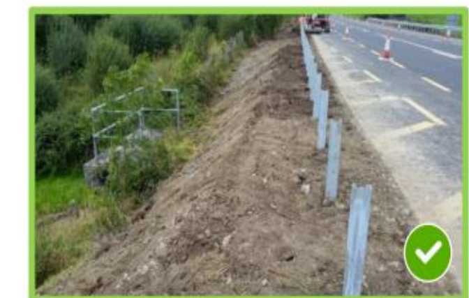
Figure 5.15 - Example of verge re-shaped and reinstated with existing topsoil
