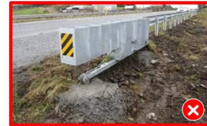
Figure 5.13 - Verge re-profiling works required at replacement terminal
